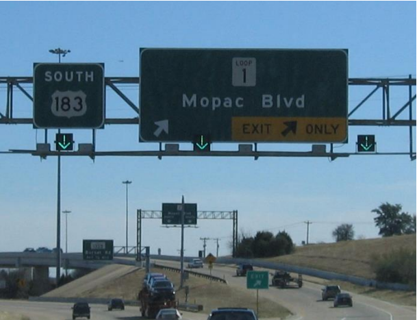
Lane Control Systems
